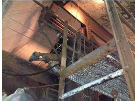
MACHINE AFTER CLEANING
